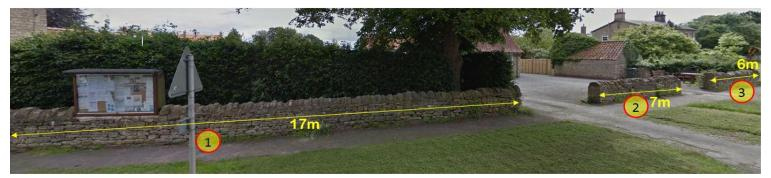
The roadside wall of the Village Hall has been gradually degrading and has now reached a state where it is in urgent need of repair and restoration. The wall would be restored to it's original state, made up of stone with concealed lime mortar, where the mortar is used to bond the stone together and is not normally visible. The work involves the replacement of all damaged stone, reversal of repairs inconsistent to the original wall and the use of lime mortar.
