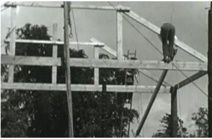
A group of men working on the construction of a Dutch barn. The wooden frame has been erected, and long ladders allow men to go up and down to fix beams that are being hoisted. Beams are lifted using ropes. No Health and Safety here!
