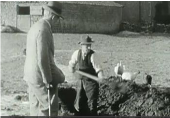
Mr Judson and a man digging drains - all by hand with the mandatory observer leaning on a cane
