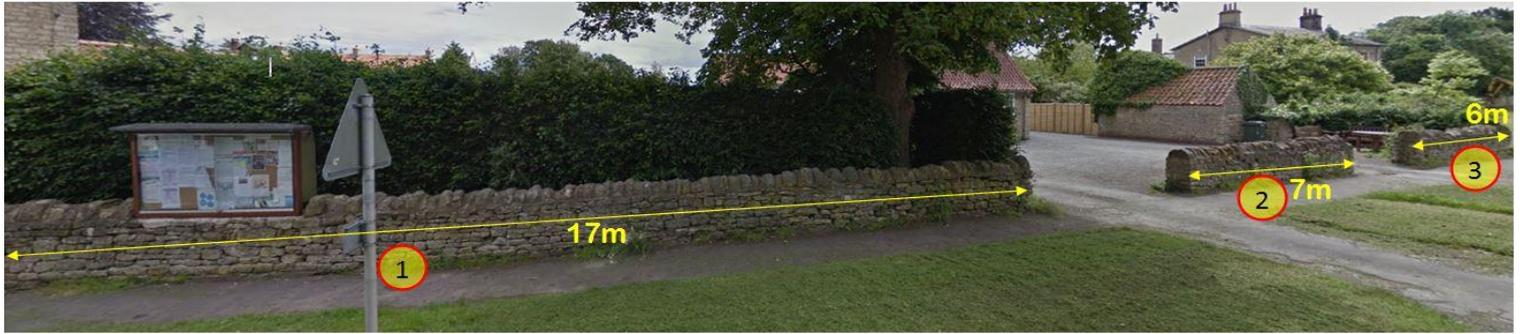
The roadside wall of the Village Hall has been gradually degrading and has now reached a state where it is in urgent need of repair and restoration. The wall would be restored to its original state, made up of stone with concealed lime mortar, where the mortar is used to bond the stone together and is not normally visible. The work involves the replacement of all damaged stone, reversal of repairs inconsistent to the original wall and the use of lime mortar.
